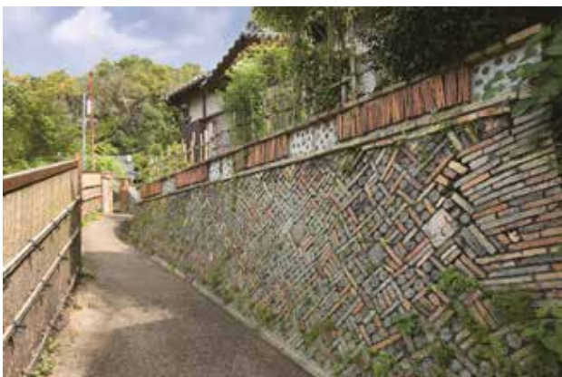
Kamagaki-no-Komichi: A path bordered by beautiful walls and fences inlaid with kiln tools arranged in a geometric pattern (Seto City)
